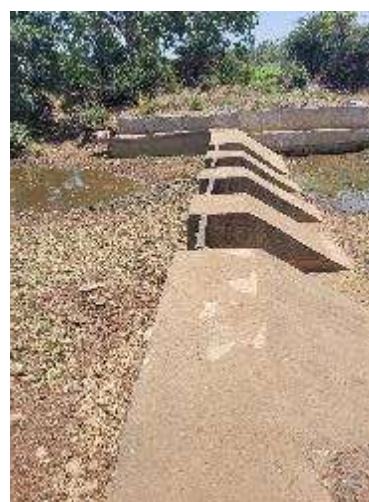
Figure 16: Stop Dam in Nagori
