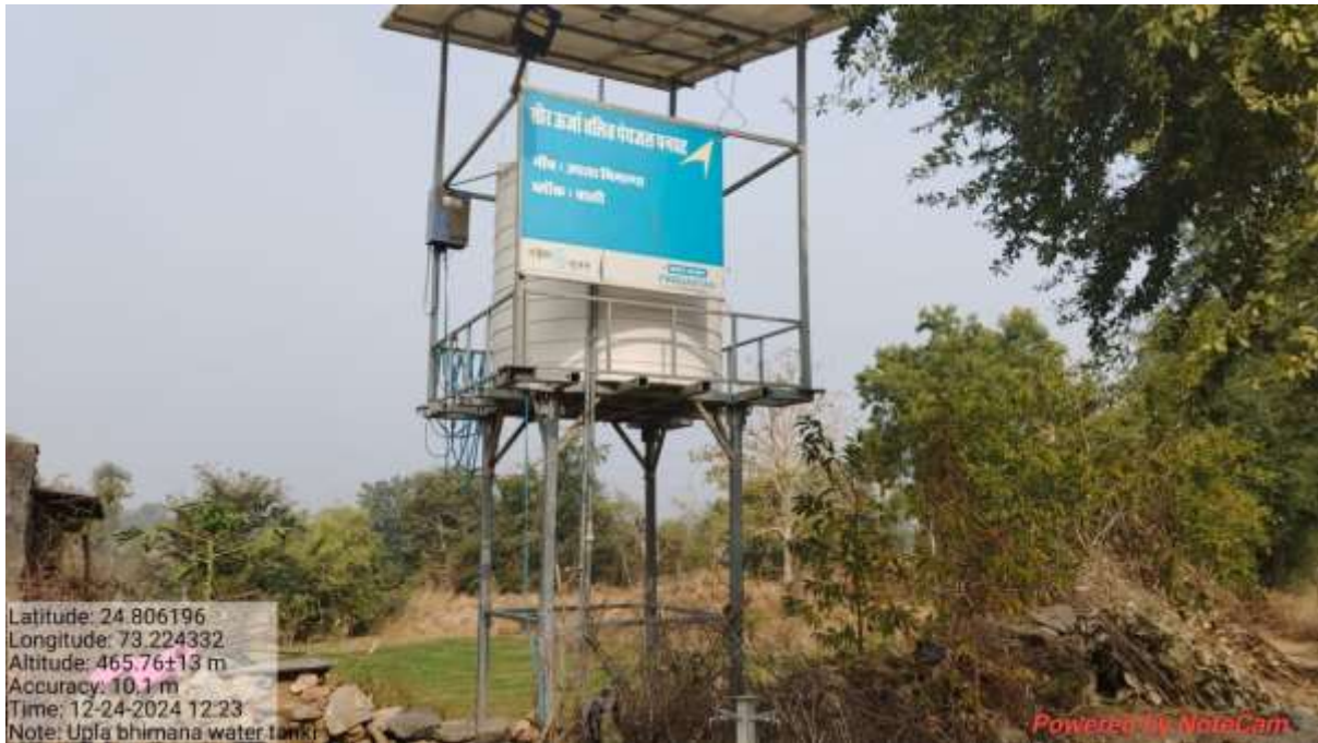
Figure 7: Community Water Harvesting Structure
