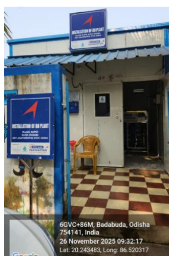
Image 1: (Above) An installed and functioning RO plant Badabuda, in Badabuda, Odisha
